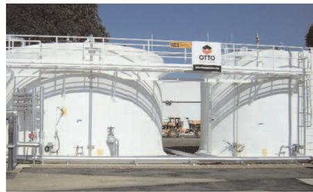
**Components for the Sacramento BioDigester (above), including pumps, valves, liquid transfer piping, heating elements and controls, were constructed on skids and brought to the site to be connected. Atlas Disposal installed a BioCNG fueling station (right) that uses biogas from the adjacent CleanWorld digester.**
