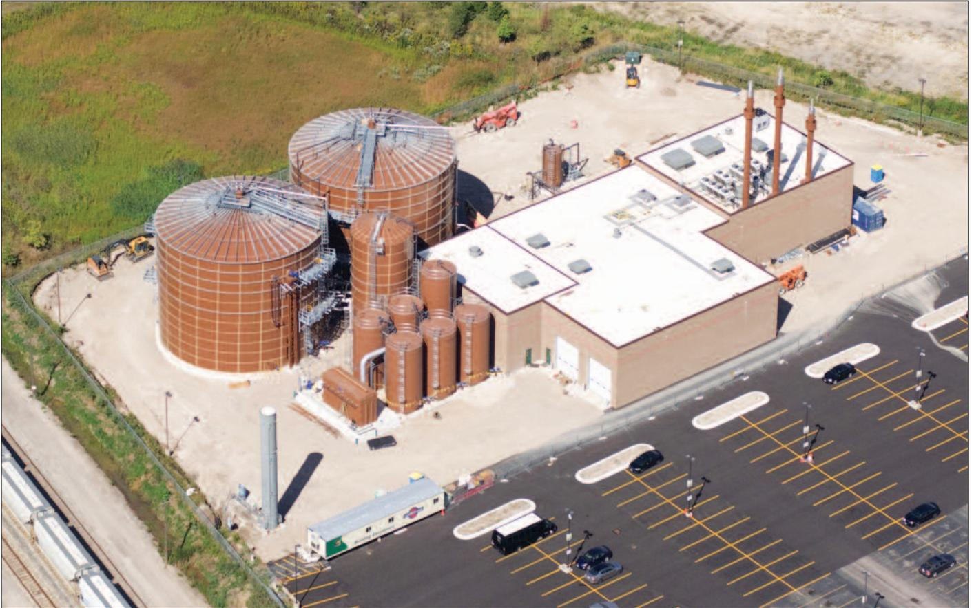
The Forest County Potawatomi Community (FCPC) committed themselves towards achieving energy sovereignty when they built a two megawatt renewable energy plant powered with biogas created by anaerobic digestion. The digesters operate on liquid (pumpable) food waste. This feedstock comes from Potawatomi Bingo Casino as well as byproducts of local and regional food processing resources.
