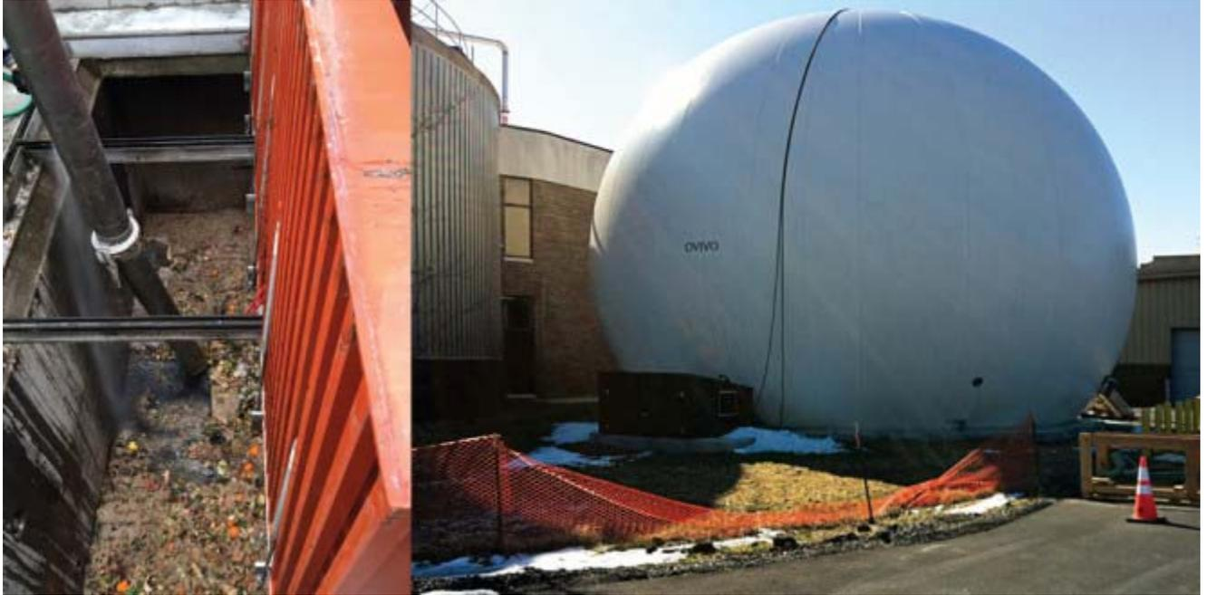
Construction of a \$3 million receiving facility for food waste and other high strength organics was completed in January (left). Biogas from the AD tanks is directed to a gas storage membrane system (right).
