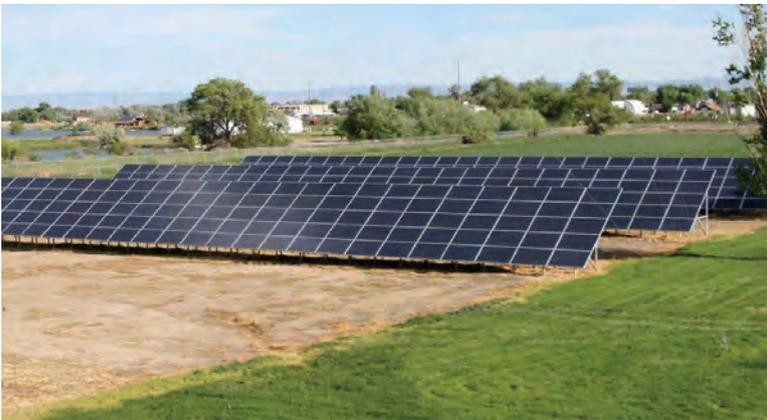
The Persigo plant also uses renewable energy with a 98 kW Sunsense solar photovoltaic system installed in 2011.
