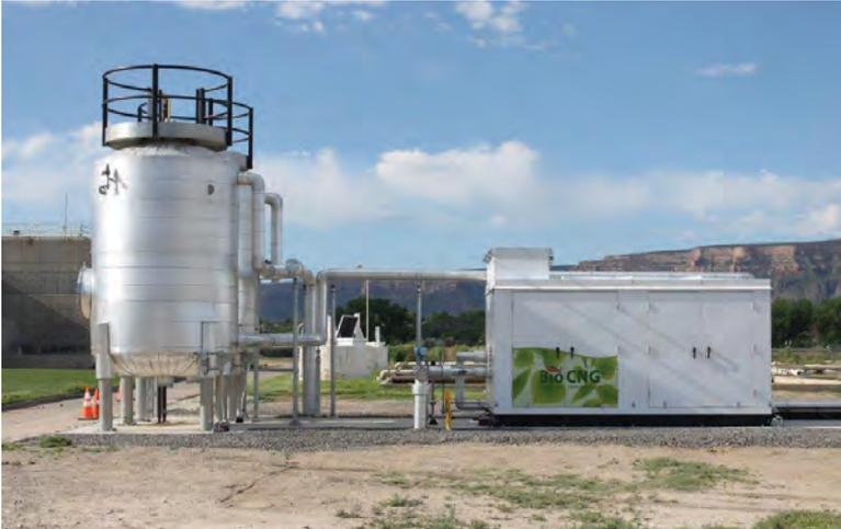
After biogas is cleaned and compressed, it is piped to a CNG fueling station so employees don’t waste fuel and time driving 6 miles to the wastewater treatment plant.
