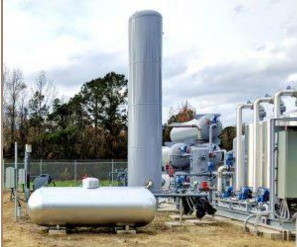
The biogas upgrading system at Optima KV consists of pressure-swing absorption to remove CO<sub>2</sub>, H<sub>2</sub>S and other constituents. Cleaned biomethane is pressurized to be sold to Duke Energy via its subsidiary, Piedmont Natural Gas. Photo courtesy of Cavanaugh
