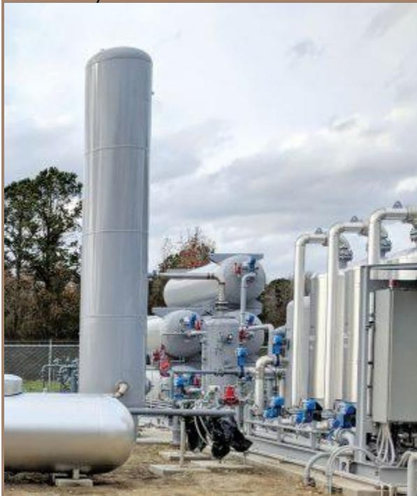
Biogas upgraded at Optima KV is cleaned and pressurized to be sold to Piedmont Natural Gas. The Optima KV project collects biogas from five digesters processing manure from 60,000 hogs. Photo courtesy of Cavanaugh
