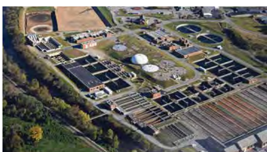
The Roanoke Regional Water Pollution Control Plant treats an average of 37 mgd.
