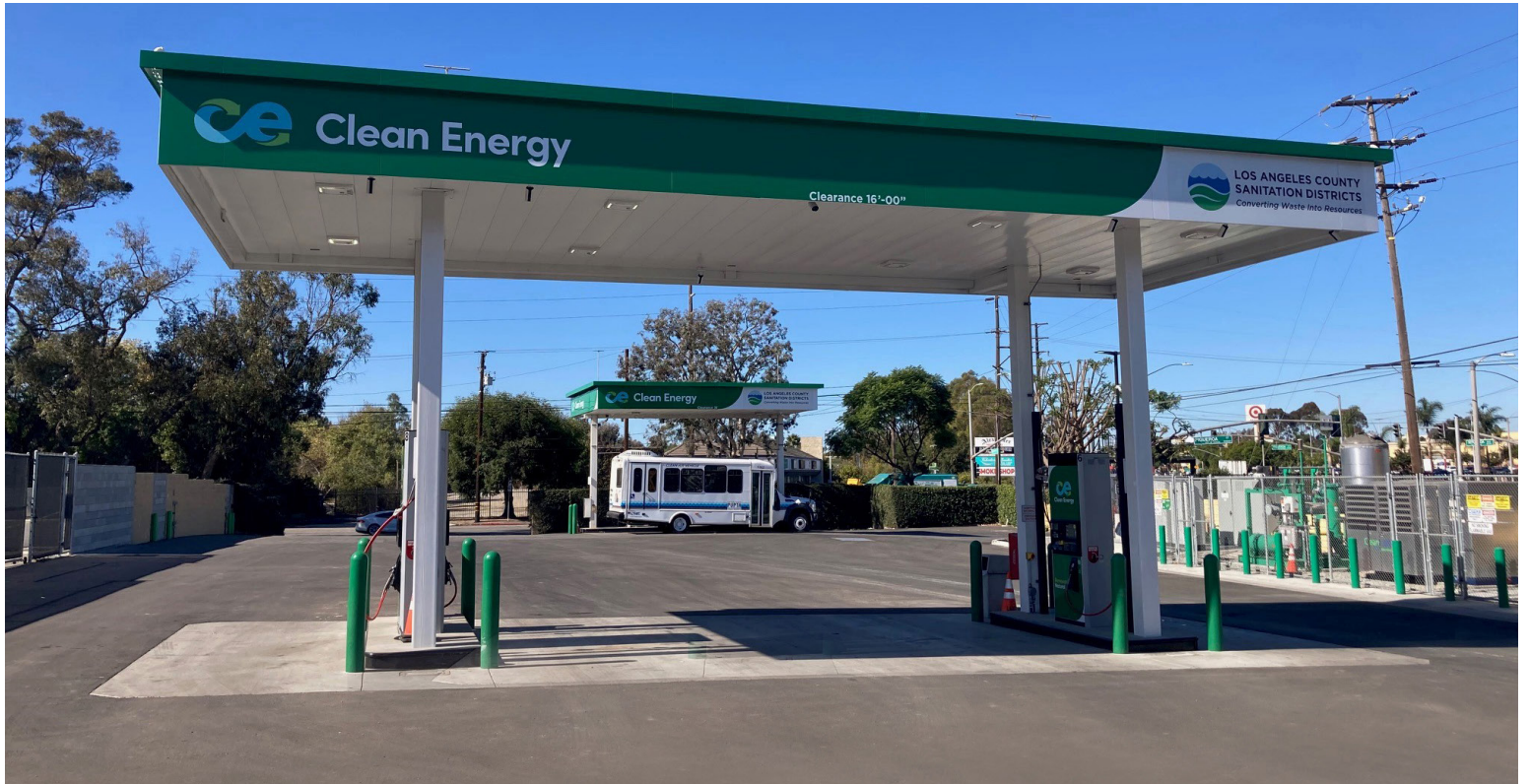
Clean Energy's expanded renewable natural gas fueling station in Carson, CA (Photo: Business Wire)
